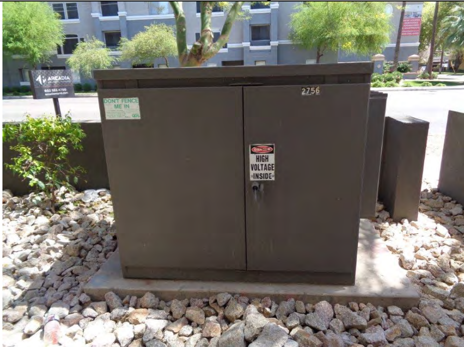
Pad-mounted transformer
