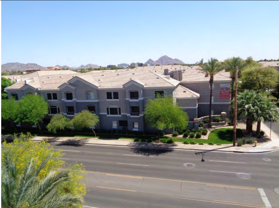
East adjacent property
