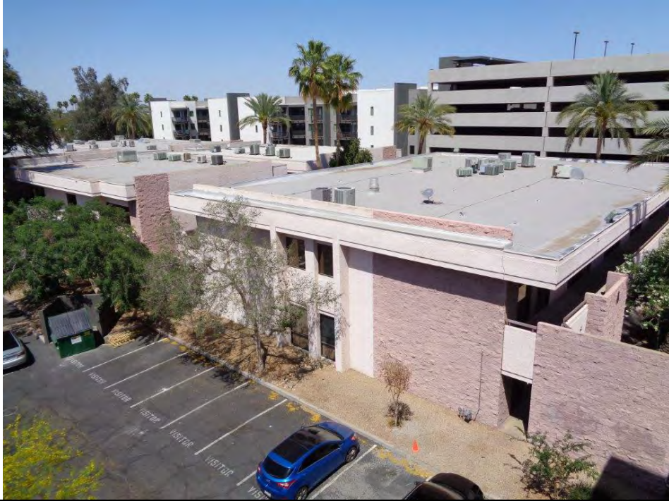
North adjacent property
