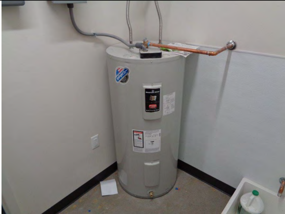
Typical electric water heater
