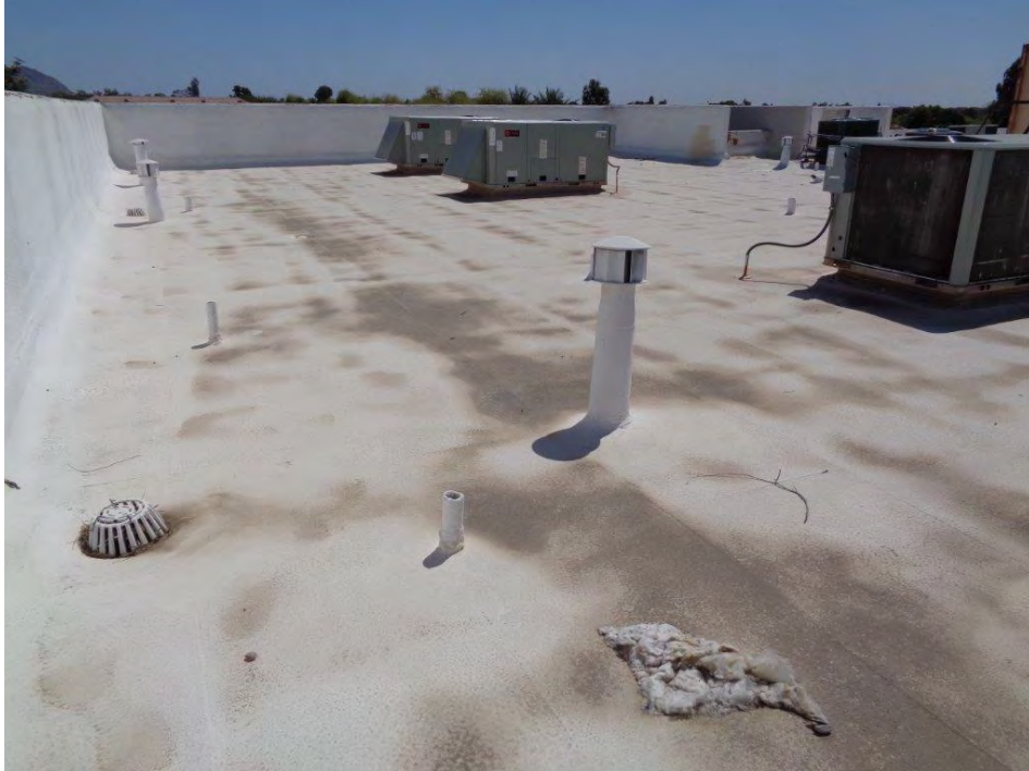
Typical roof surface
