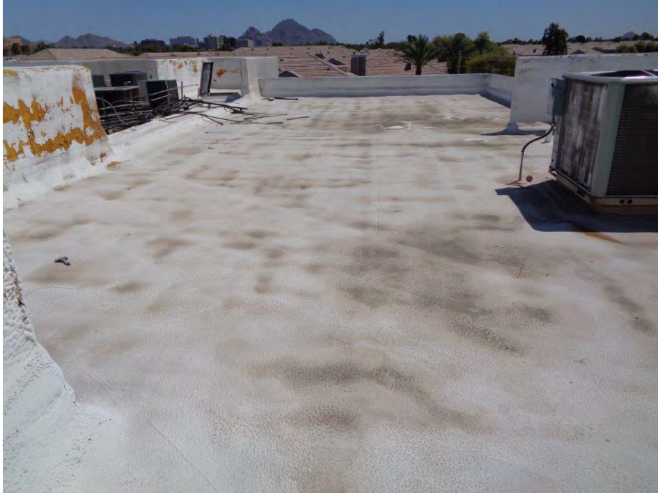
Typical roof surface
