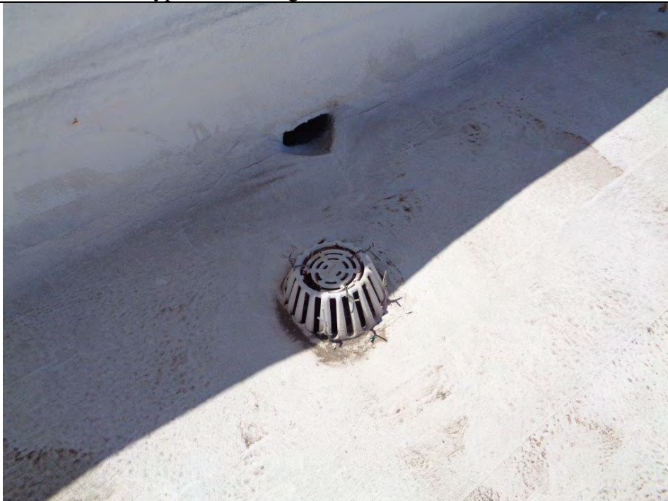
Typical roof drainage
