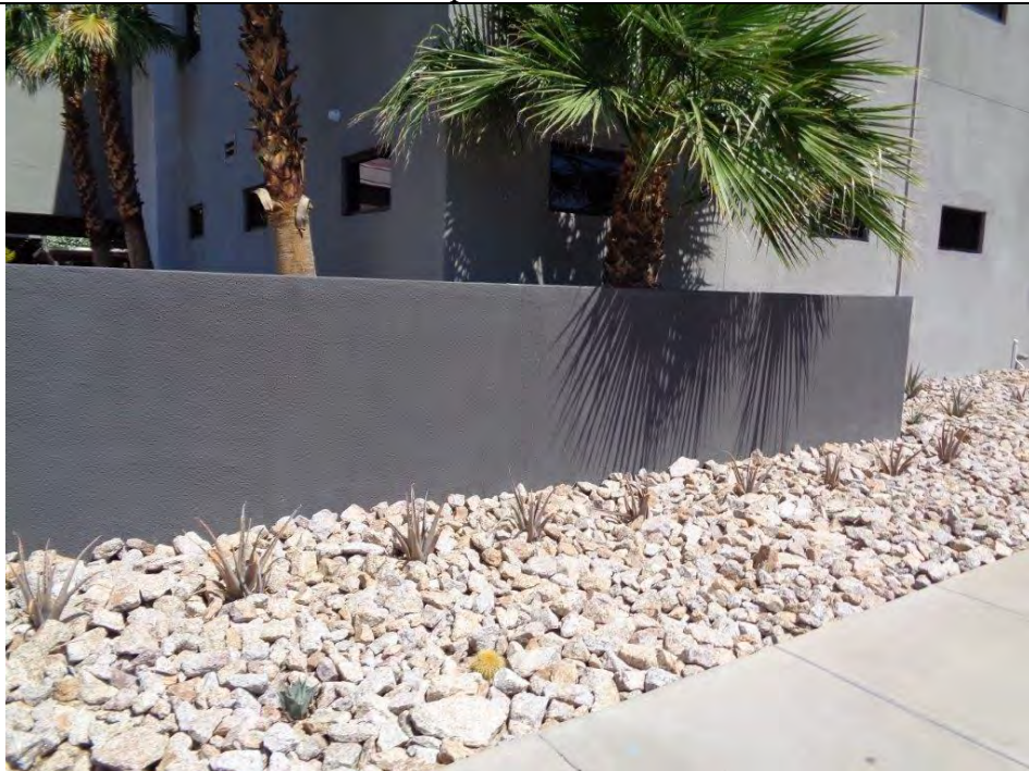
Perimeter wall along portion of southern boundary
