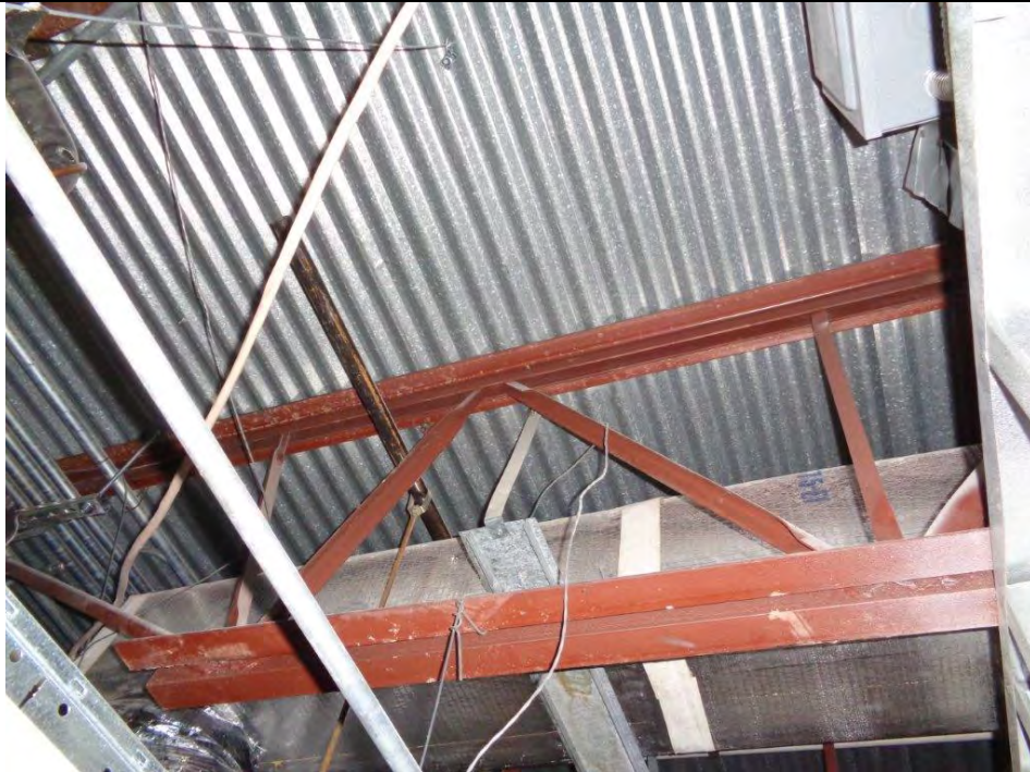
Steel framing and floor decking
