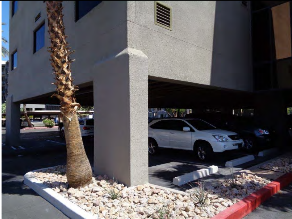
Concrete column supporting tuck-under parking area
