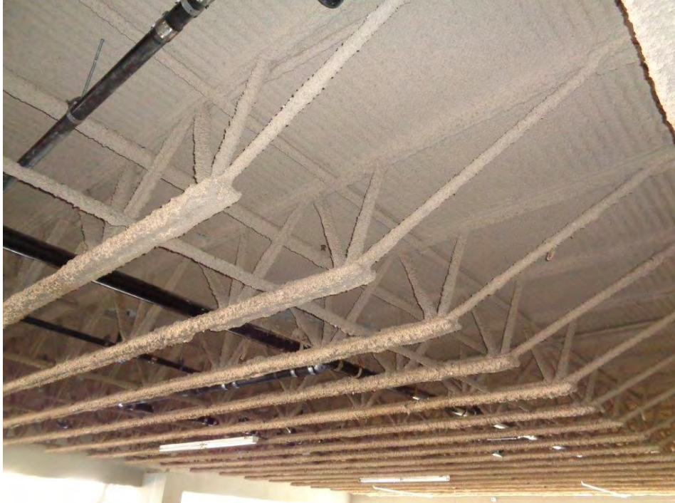
Steel joists and floor decking at tuck-under area
