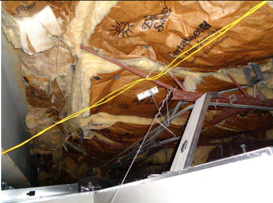
CMU wall, steel framing and roof decking
