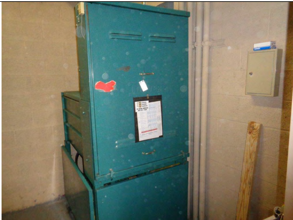
Elevator equipment (original)
