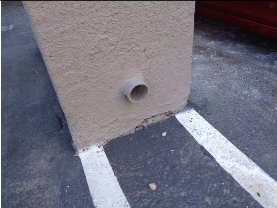
Roof drainage to asphalt
