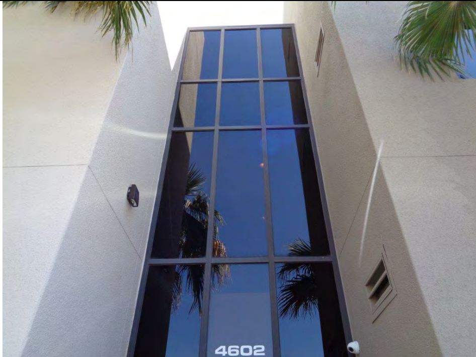
Curtainwall at western boundary of structure
