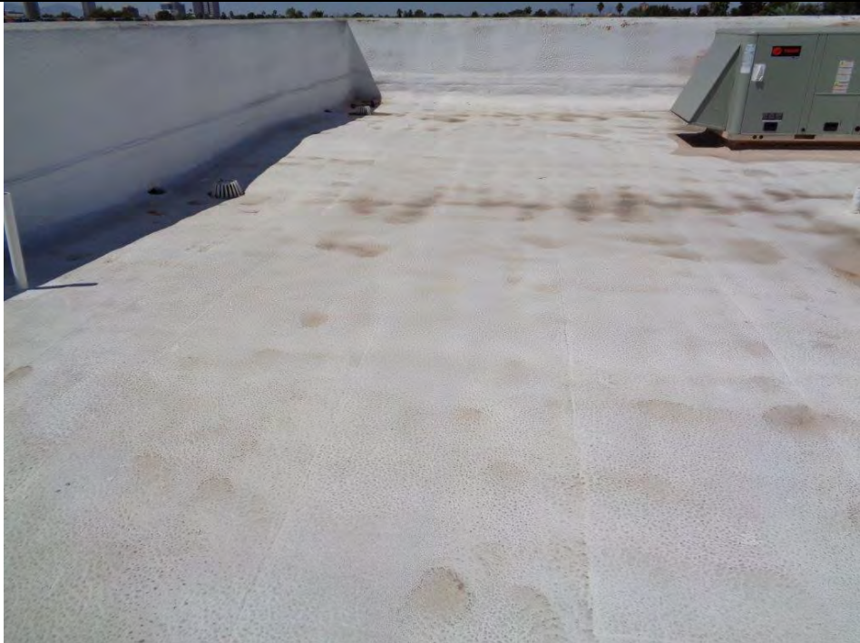
Typical roof surface
