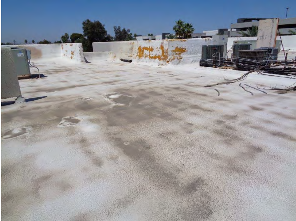
Typical roof surface
