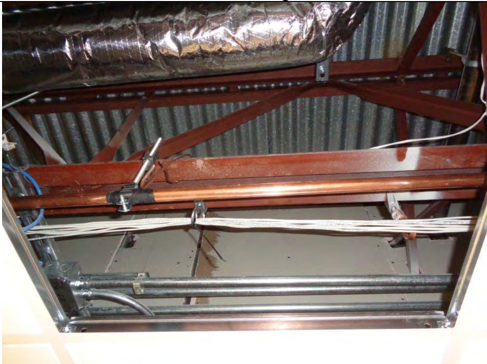
Steel framing and floor decking
