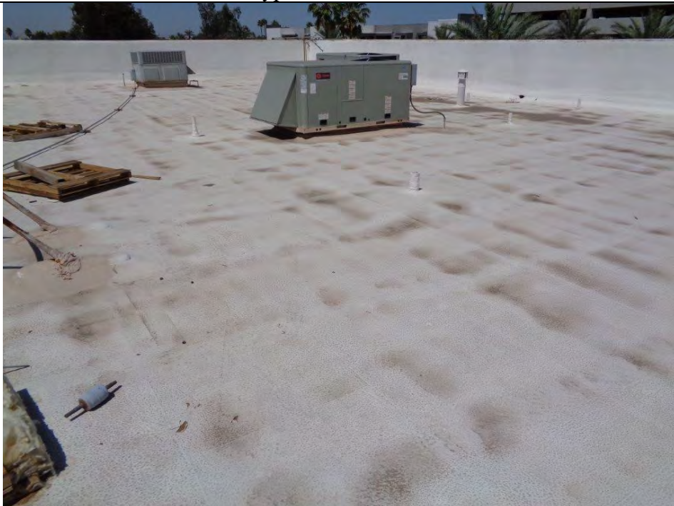
Typical roof surface
