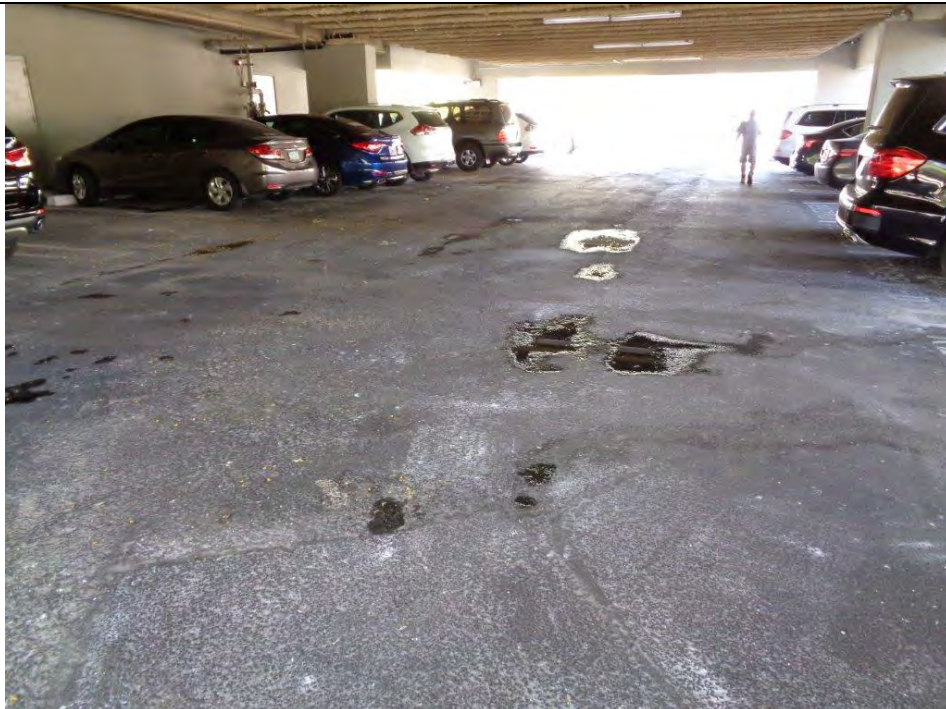
Typical asphalt pavement at tuck-under area
