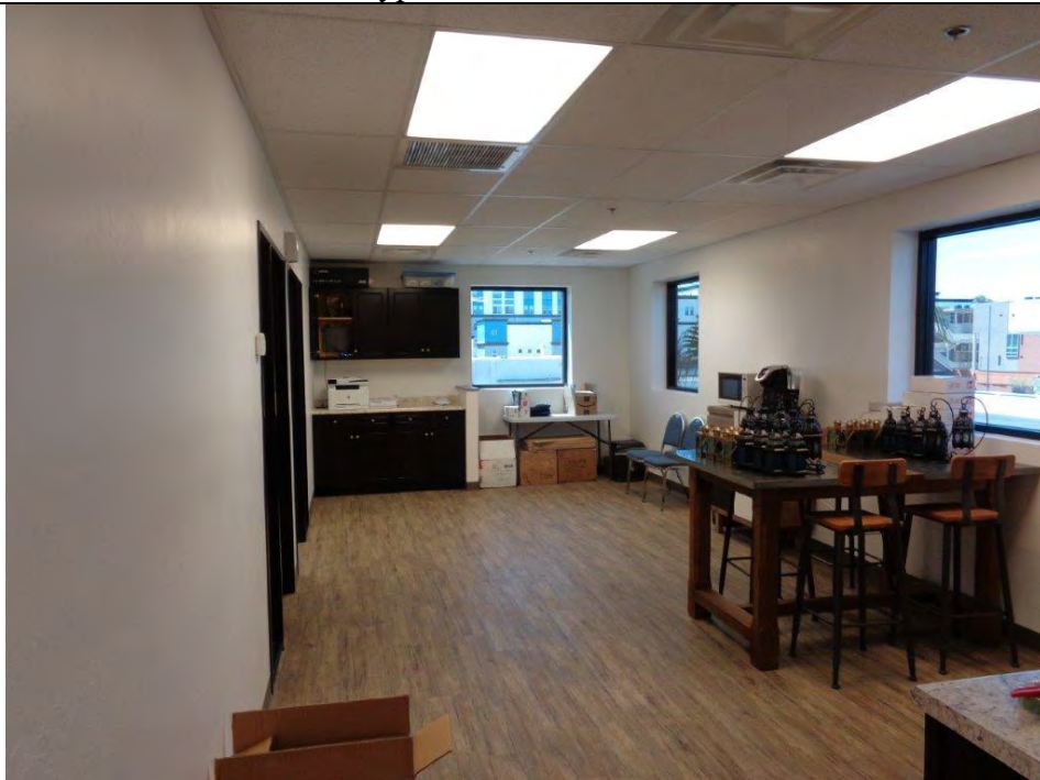
Typical interior finishes
